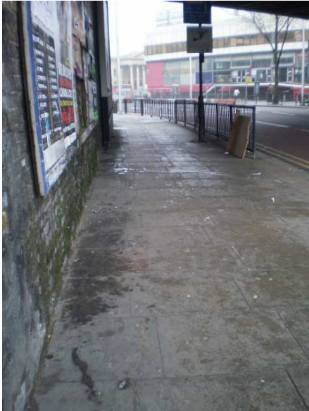
Under Railway Bridge - Western side of Walworth Rd
