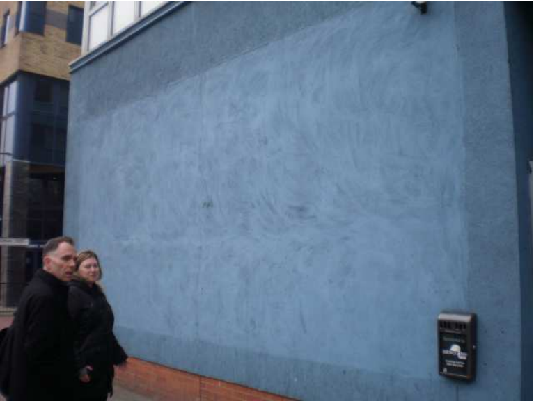
(Back on the Walworth Rd) Dead frontages to Julian Markham House.
