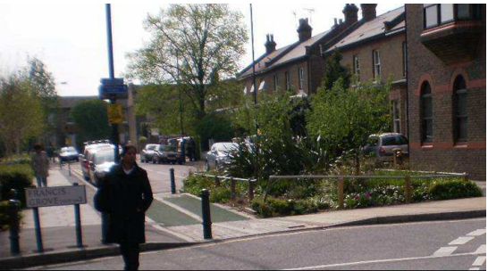
Planted road closure (with cycle access) between main road and residential street in Wimbledon
